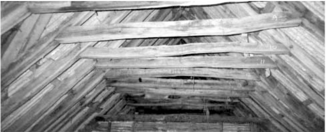
**Illus 3** General view of the roof, showing the sequence of contemporary carpenter's marks on the collars.
