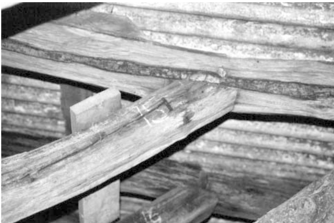
**Illus 6** *The carpenter's mark on BR15C. The strips of bark on each corner of BR15RE are visible behind.*
