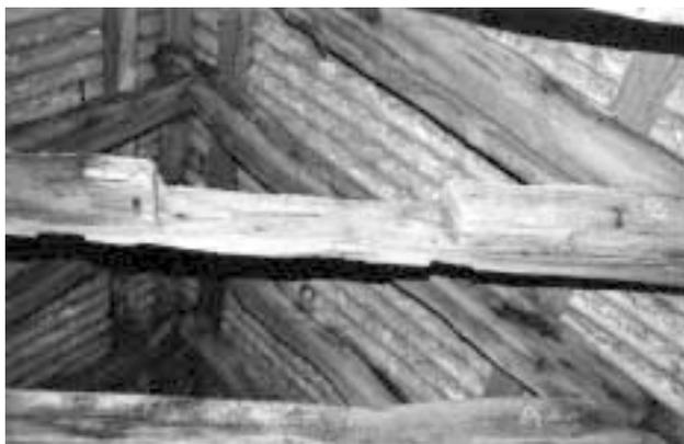
**Illus 11** BR8C, showing a large notch cutting House 2 carpenter's marks, which lie just to the left of the notch. The redundant pegholes on the underside of the collar are also visible.
