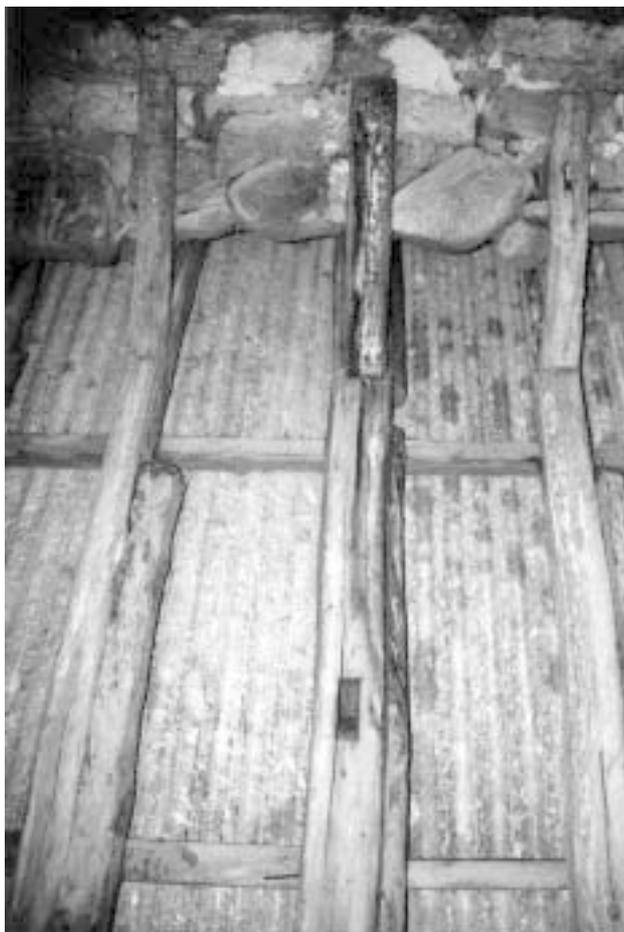
**Illus 10** Redundant mortice in BR3RE; the sloping face of the mortice lies to the top of the joint. The ashlar post-construction of House 2 can be clearly seen.
