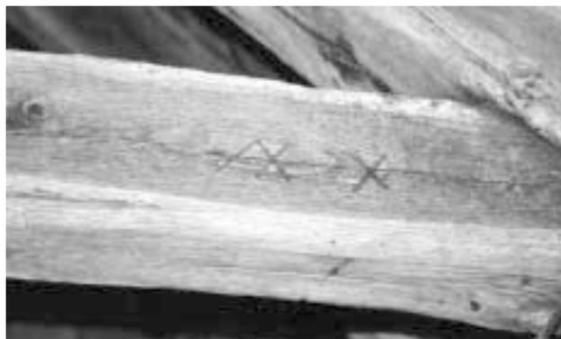
**Illus 12** Carpenter's marks on the north face of BR6C. The sapwood on the corners of the boxed heart baulk is clear.
