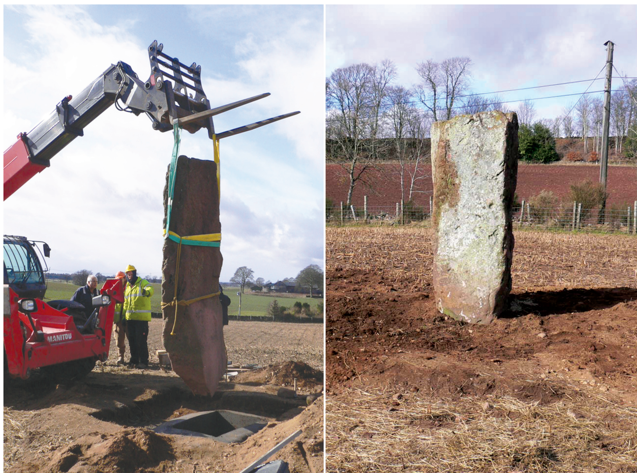
Illus 6 The re-erection and the final position of the stone.
