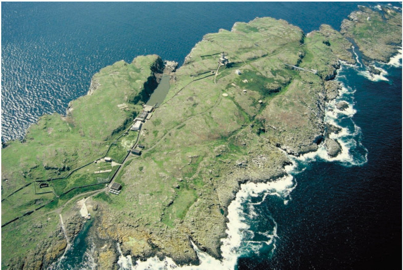
1 The landscape of the island is now dominated by the infrastructure of the Northern Lighthouse Board – with the Stevenson light top and centre. The monastery is at the lower left. (© Fife Council)
