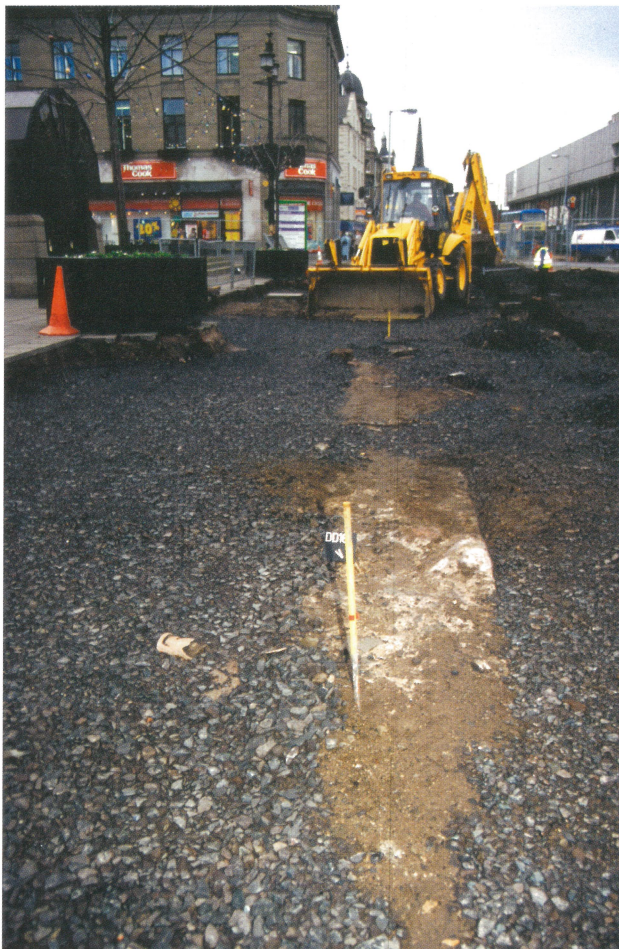
Plate 2 The foundation wall of the Pillars uncovered during environmental improvements in the city centre, towards the west (© SUAT Ltd)
