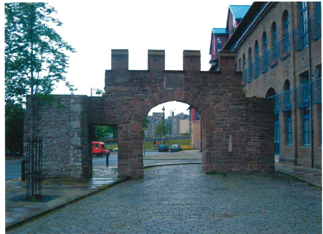
Plate 6 Wishart Arch from the east, in 1989 before restoration (top) and today after restoration (bottom). (© SUAT Ltd)
