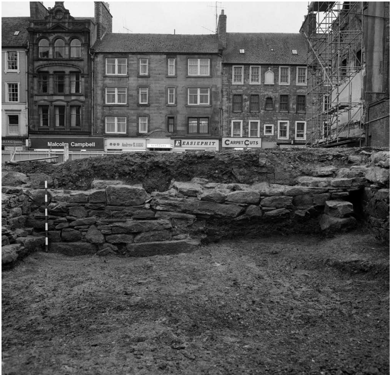
Illus 97 South Sector: west end of south wall (Wall 2020) of 'Old Parliament House'/Masonic Hall (Building G), showing two phases of construction, looking south. (© Courtesy of RCAHMS. Licensor www.rcahms.gov.uk )
