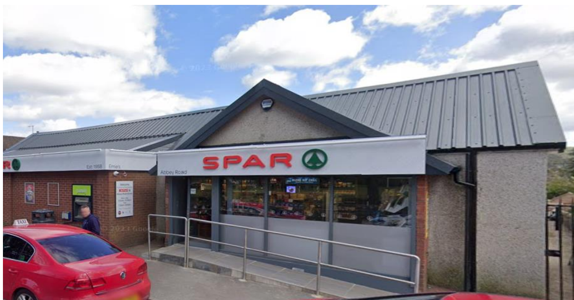
Scone SPAR shop with its new roof. Image courtesy of Google Streetview.
