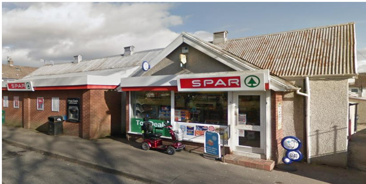
Scone SPAR shop prior to recent re-roofing. Image courtesy of Google Streetview.
