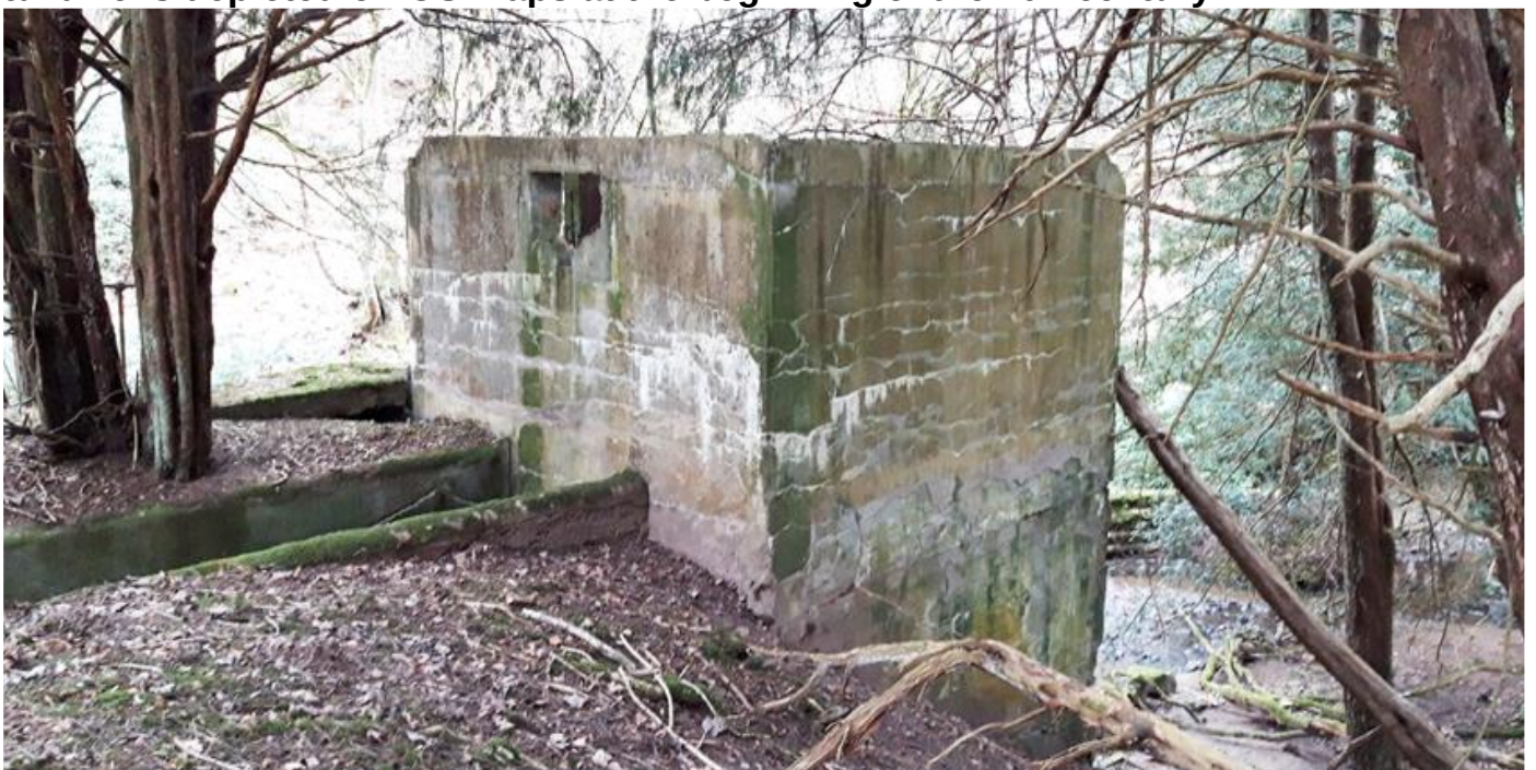
A view from the NNE of the 'Powerhouse' at the WSW end of the reservoir. Water to power the turbine entered the turbine chamber via a concrete channel (centre left of image and bottom left image on the next page). Images copyright: J Sherriff.
