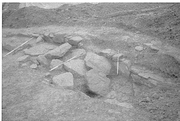
Illus 15 The collapsed roof in the main chamber.
