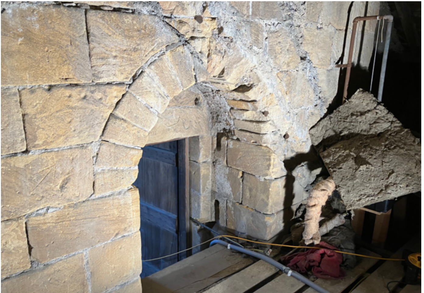
Upper portion of door linking tower and nave viewed from upper chamber. Image copyright B Manson.
