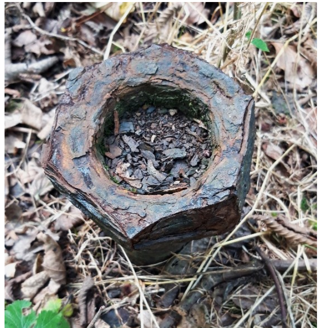
A view of the holdfast of the northeasterly of the pair of 9.2-inch guns at Braefoot. Most of the steel bolts which secured the gun mounting are still visible – some retaining their nuts. The image on the left shows one of the lockers in which ammunition was stored in readiness.
