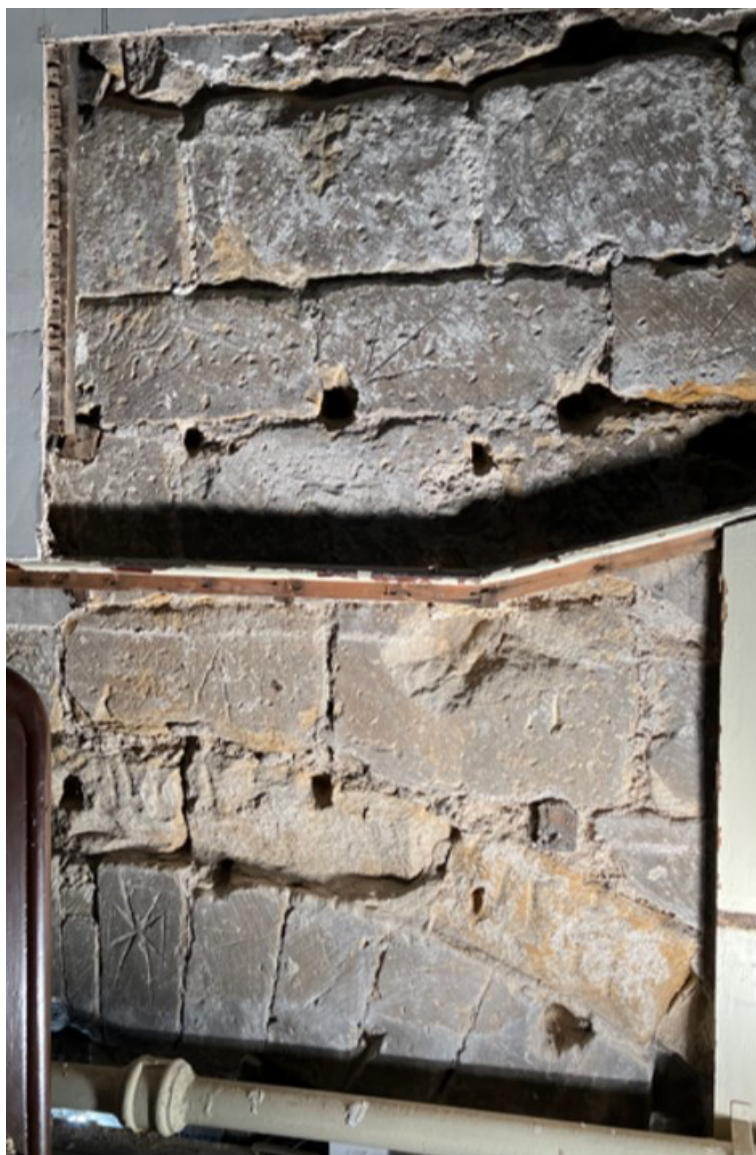
Top of great western arch and lower portion of upper doorway linking nave and tower. Image: B Manson
