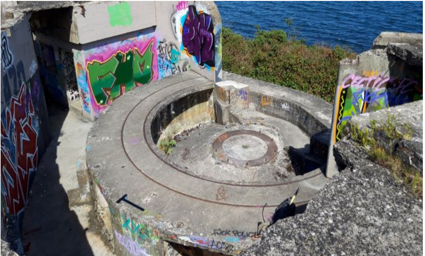
A view down into the gun-pit of the battery on Charles Hill, Aberdour. A twin 6-pounder gun was installed here at the beginning of World War Two as a defense against rapid-moving enemy vessels such as motor torpedo boats.
