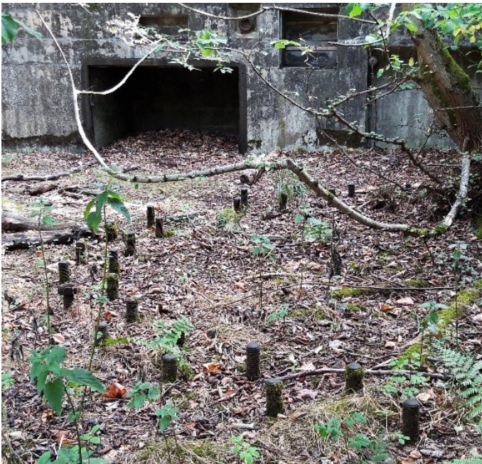
A view of the holdfast of the northeasterly of the pair of 9.2-inch guns at Braefoot. Most of the steel bolts which secured the gun mounting are still visible – some retaining their nuts. The image on the left shows one of the lockers in which ammunition was stored in readiness.
