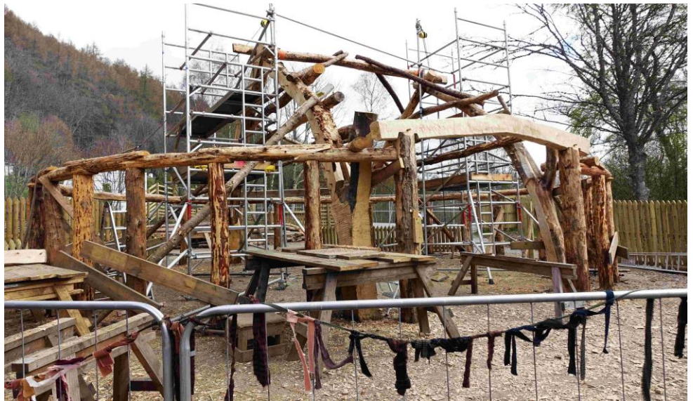
Above: a roundhouse under construction showing timber frame.
