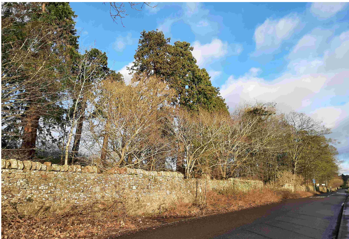
A view of the wall that marked the outer limits of the Rossie Priory Estate on its S. Image copyright: LM Thoms.
